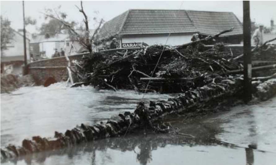
The bridge acted as a dam until it burst.
